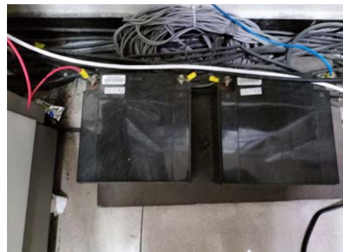
Batter Back Up ตู้ PPS 12V 26AH = 2 ea
